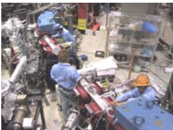
FIGURE 6. Installation of the beam duct for the multi-pole magnets
