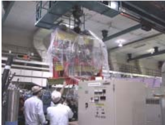
FIGURE 8. New In-vacuum undulator being transported in the storage ring room
