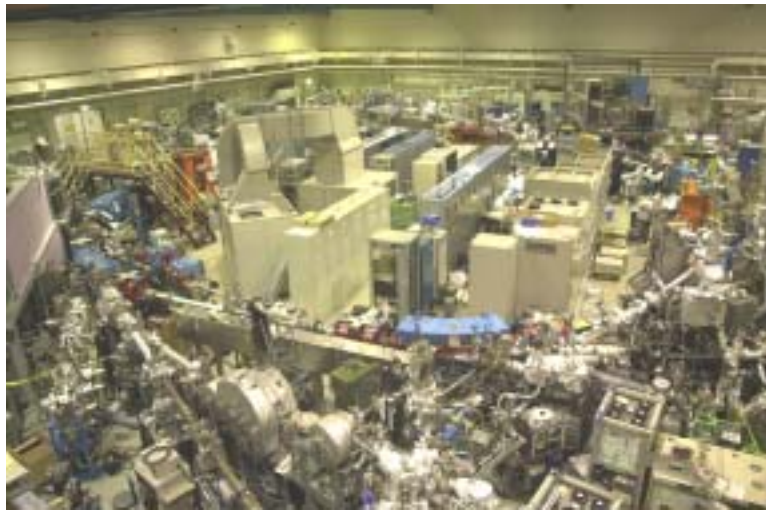
FIGURE 14. UVSOR-II just after finishing the installation
